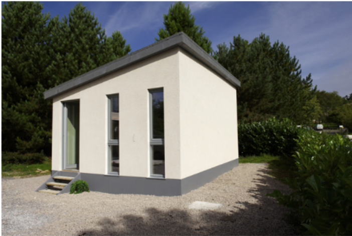
Fig. 1. The completed HempPod building at The University of Bath.
